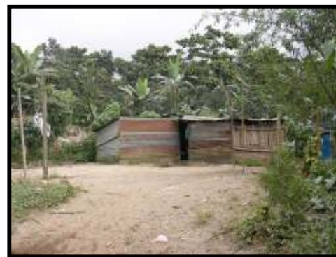
Displaced labourers often find themselves and their families living in a "ranchito" constructed from corrugated sheet metal, wood and cardboard. This dirt-floored shack starts as temporary but often becomes their permanent housing.
